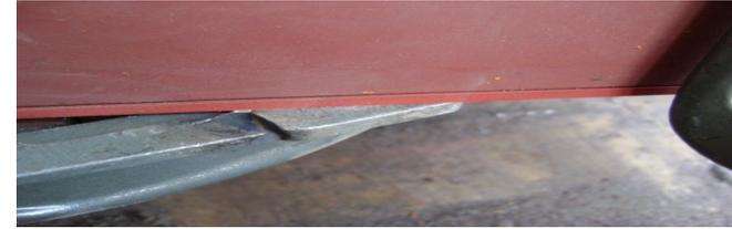
Once the assembly is tack welded and tested, continue by fully welding in the holes. After the assembly cools go back and grind the welds flush.
