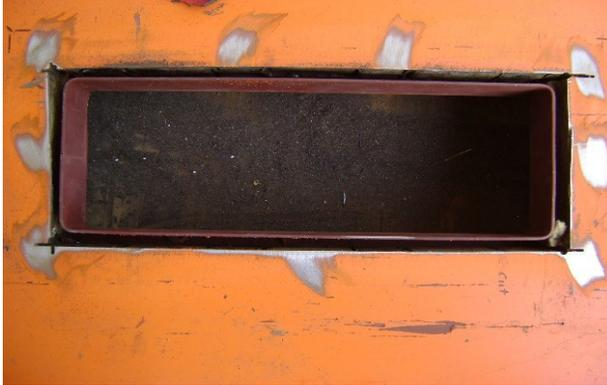
After the prep work is completed, align and tack weld one side of the assembly to the door. Flip the door and start on the other half of the assembly.
